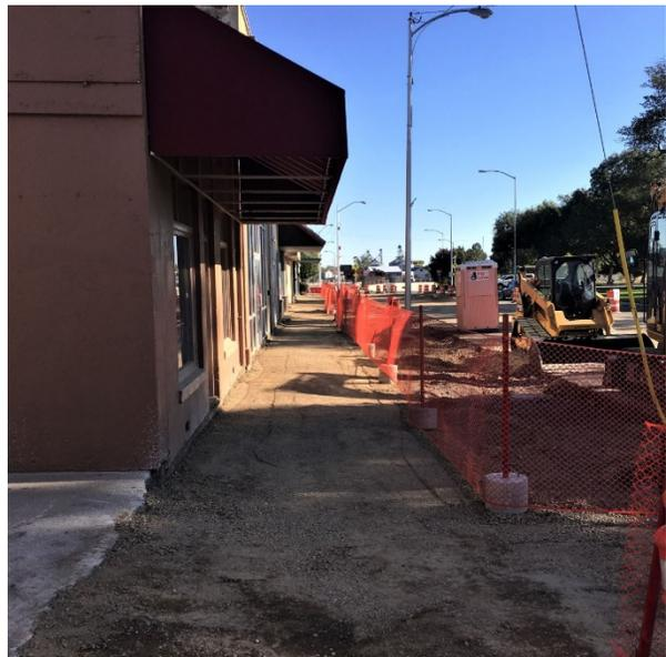
Sidewalks along Main Street have begun the demolition phase, beginning with the first block between East Jackson Street and East 2nd North Street. The first block now has a temporary, ADA compliant, compacted gravel sidewalk 6 feet out from the building face. Crews have also finished the demo of the sidewalks to the curb and have separated the sections by an orange safety fence to delineate pedestrian walkways with work areas.
